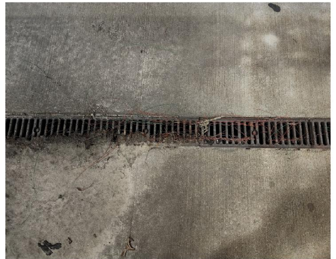
Trench Drain Grate Partially Covered with Debris
